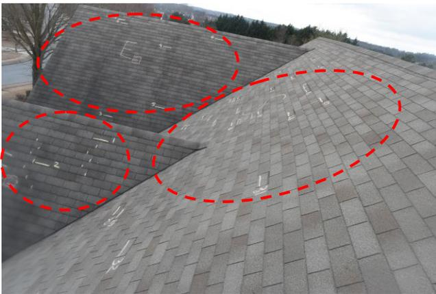
**Figure 1: DAMAGE IS PRESENT ON ALL SLOPES.**
