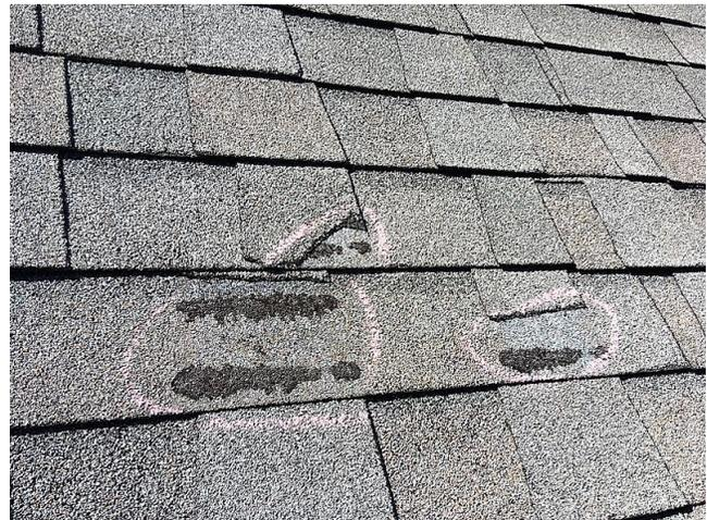
**Figure 4: TOTALLY, PARTIALLY AND DIAGONALLY TORN SHINGLE TABS.**
