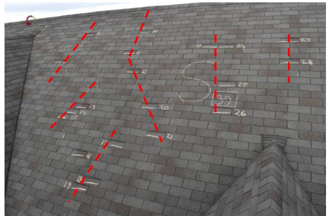
**Figure 2: DAMAGE IS CONCENTRATED ON FIELDS & FOLLOWS A PATTERN.**
