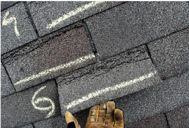
**Figure 3: SHINGLE TABS WITH DOUBLE CREASES.**
