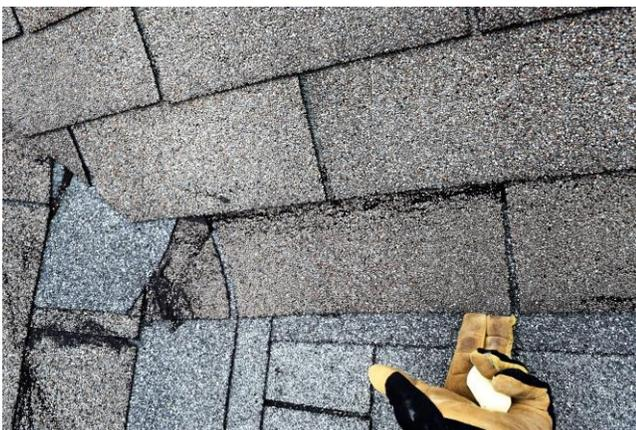
**Figure 5: CREASED SHINGLES THAT GOT REPAIRED ARE NOT SUSCEPTIBLE TO WIND DAMAGE.**
